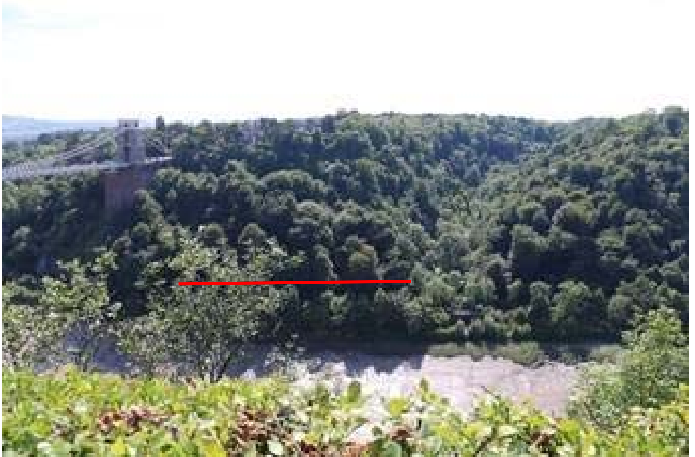
Photograph 3 – Rockfall barrier 3 location (78m long)
