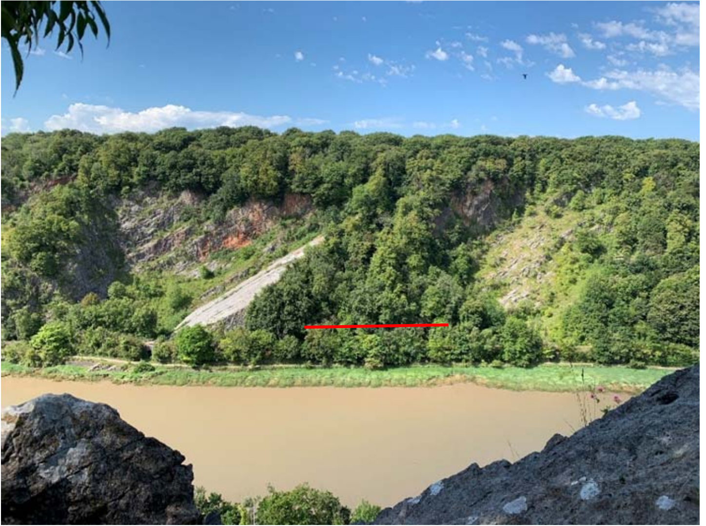
Photograph 2 – Rockfall barrier 2 location (52m long)
