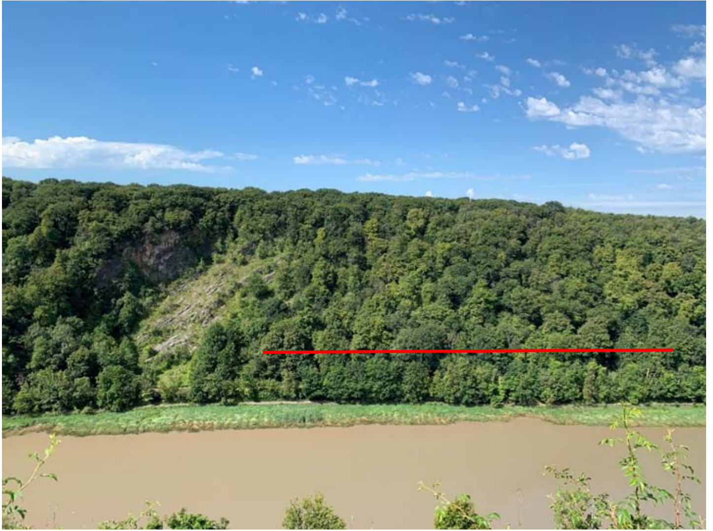
Photograph 1 – Rockfall barrier 1 location (147m long)
